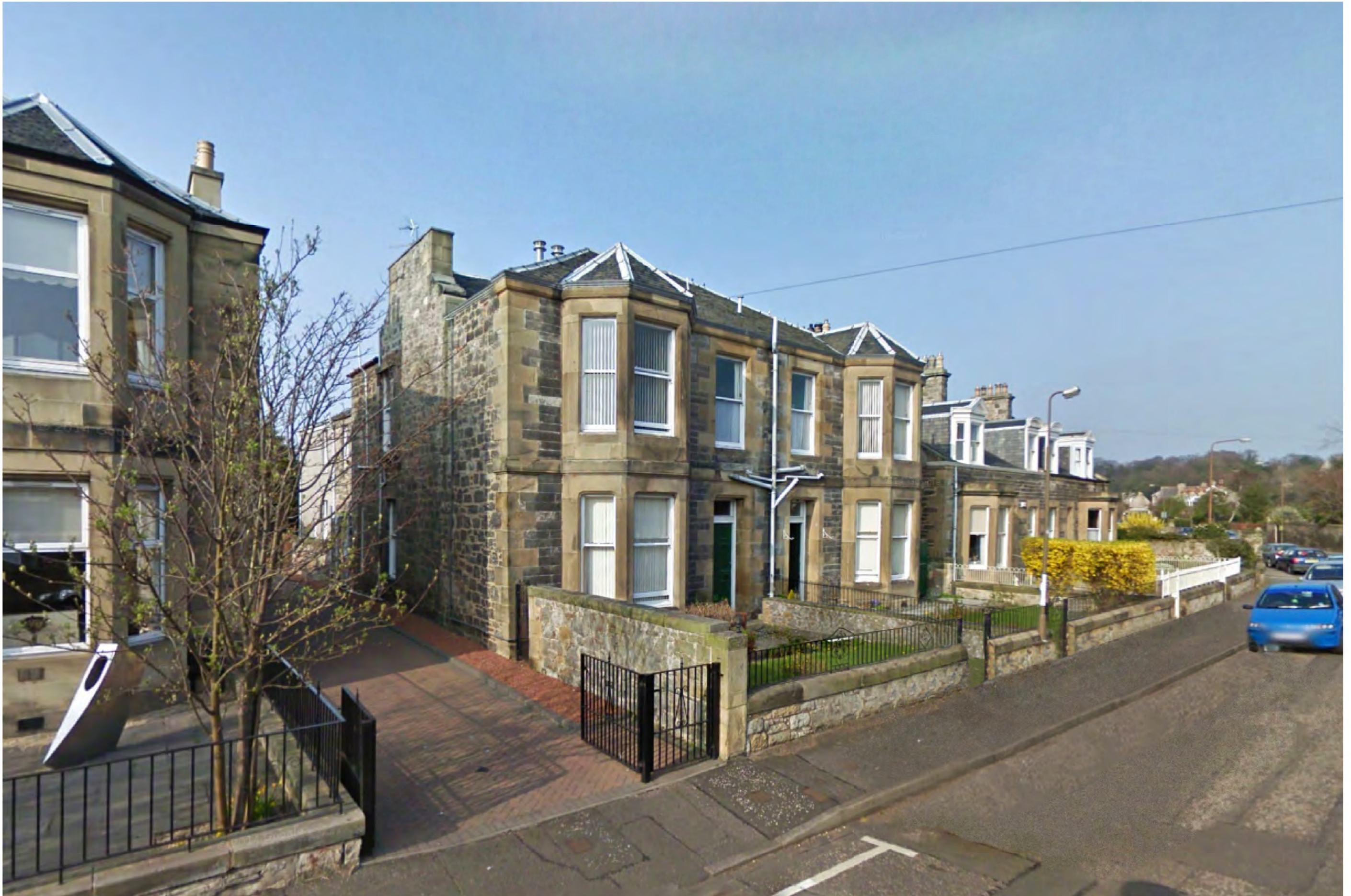
LEVENHALL FRONT VIEW 1
