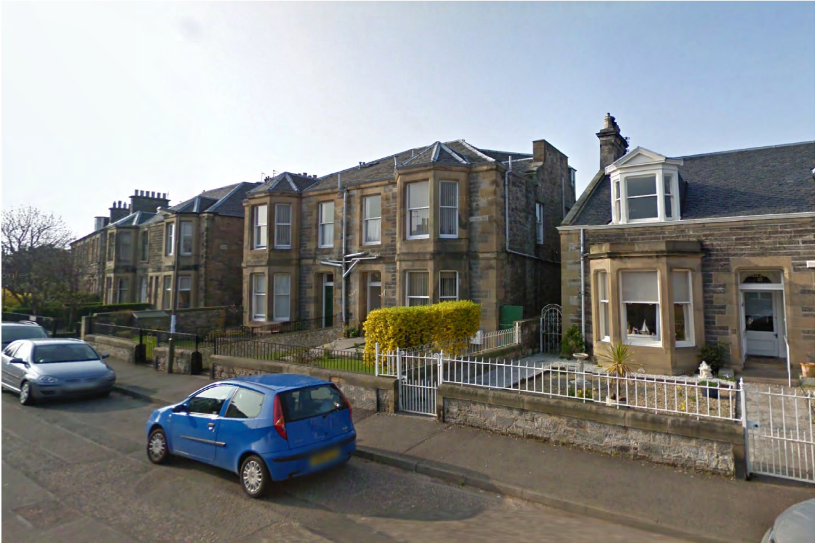
LEVENHALL FRONT VIEW 2
